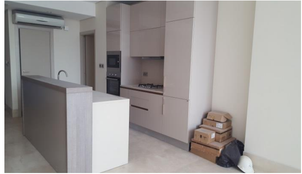
Kitchen Cabinetry – work in progress
