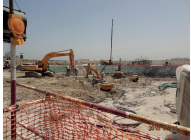
At this stage in the construction lifecycle the major ongoing works continue to center on the excavation, cutting and testing of existing piles, de-watering works and the casting of new piles for all three zones of the project construction site.
