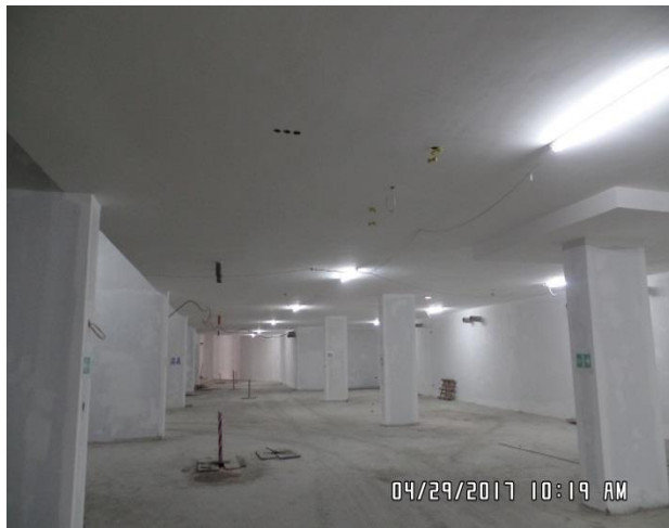
Basement – completion work in progress
