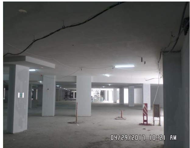
Basement – completion work in progress
