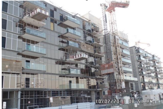
Curtail Wall Glass Façade
