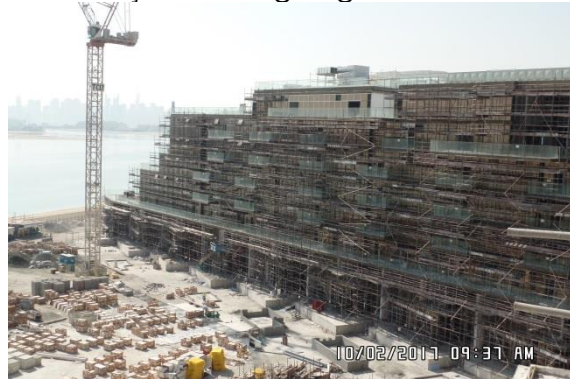
Glass Façade - Ongoing Work
