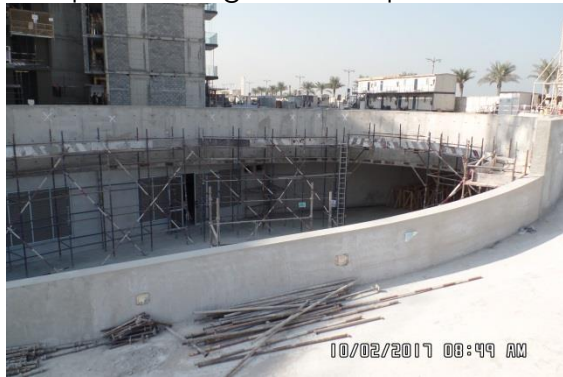
Ramp to Underground Carpark
