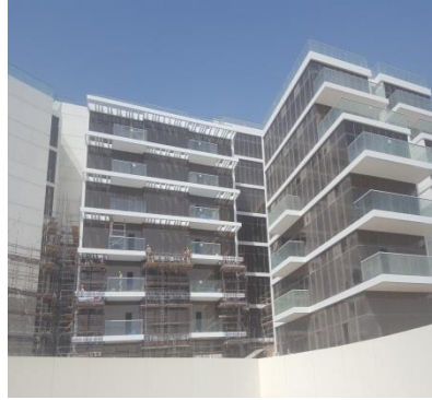
External finishing work
