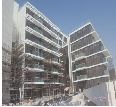
External finishing work
