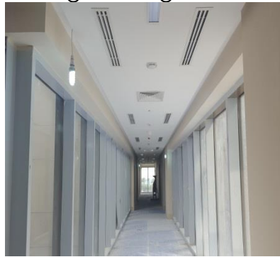
Ceiling finishing work
