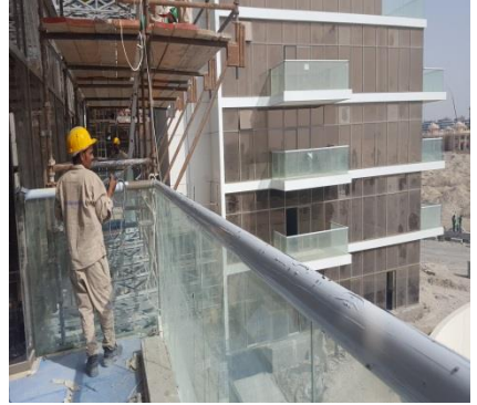
External finishing work
