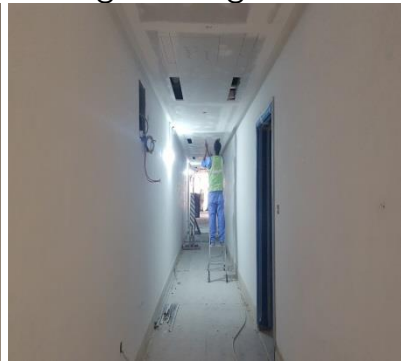
Ceiling finishing work
