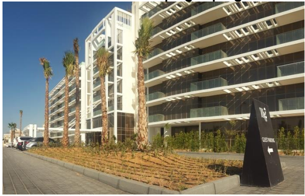
Front elevation – landscaping in progress
