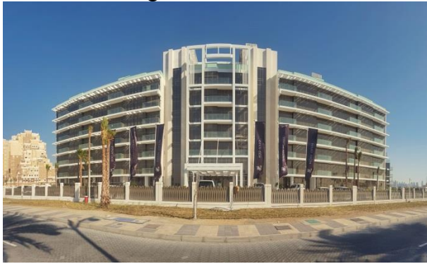
The8 - hoarding removed
