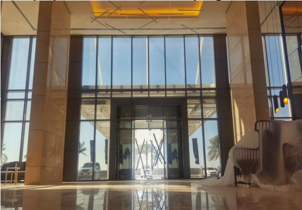
Lobby - protection removal in progress
