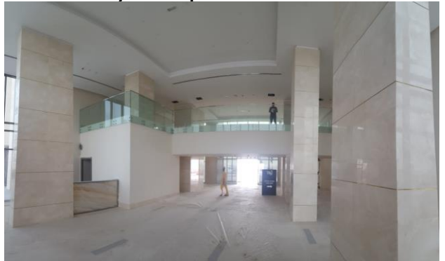
Block B lobby – with protection
